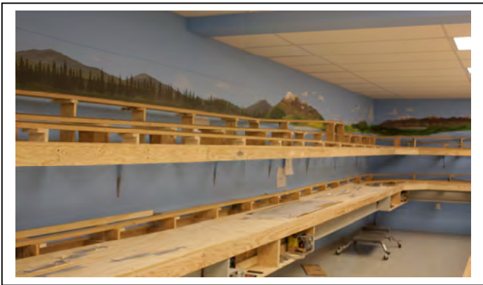
View looking south along east wall
